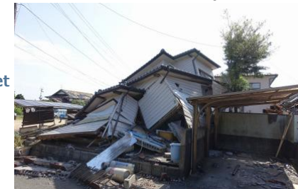
A wooden house built to the pre-2000 standards that collapsed due to the Kumamoto earthquake
