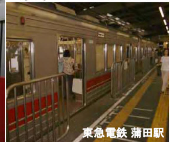
Fixed Platform Fence
