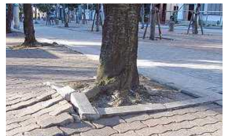
Uneven sidewalk due to rising tree roots
