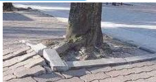
Uneven sidewalks due to roots rising out of the ground
