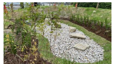
Demonstration experiment being conducted on a rain garden (Öjima-Komatsugawa Park)
