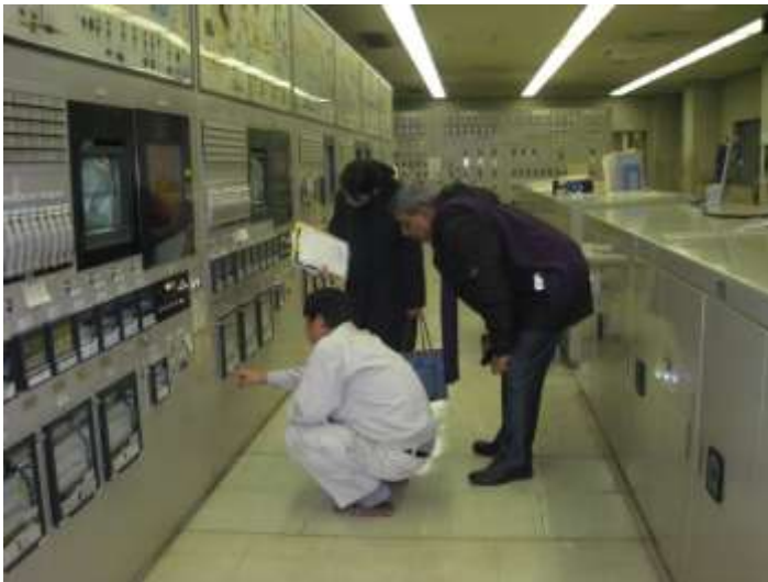
Inspecting the reading
